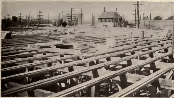
FLOOR FORMS UNDER CONSTRUCTION
